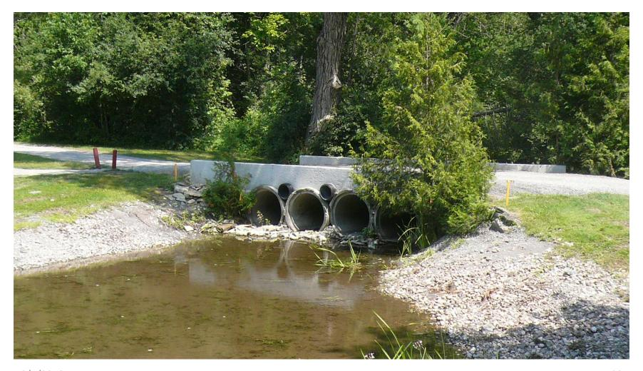
Picture 22 - Repaired right-hand cart path on the 1<sup>st</sup> hole over culverts with additional culverts installed – July 26/19
