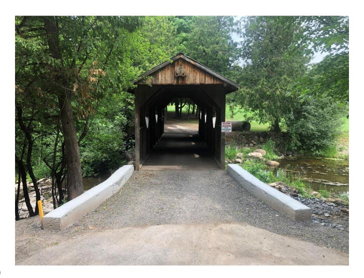
Picture 36 - West cart path approach to the covered bridge on the 5<sup>th</sup> hole with new support structure and additional culverts – July 11/19
