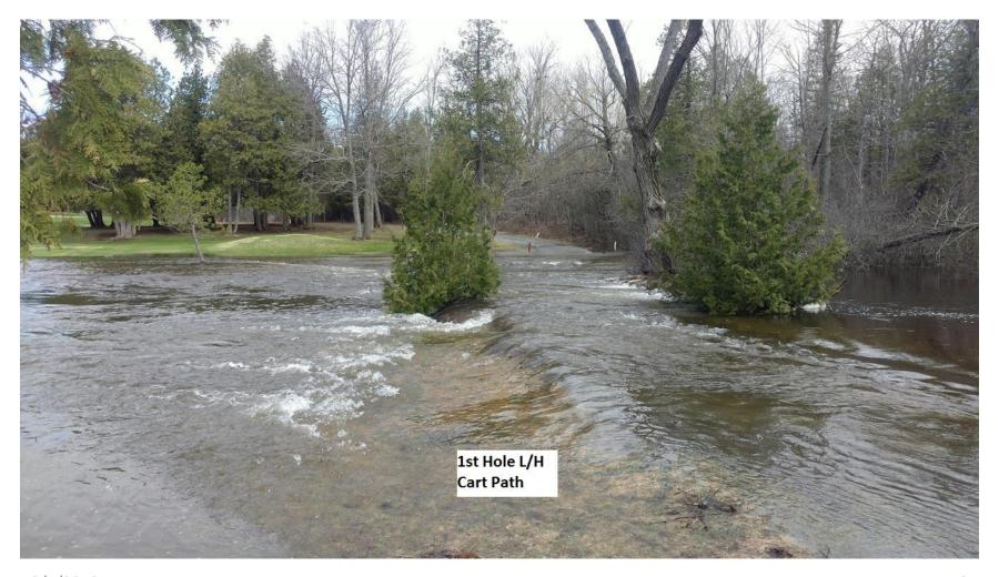
Picture 19 - Washed out 1st hole right-hand cart path over culverts - May 04/19
