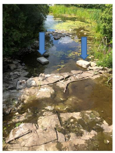
Picture 34 - Washed out concrete support slabs from the covered bridge - July 24/19
