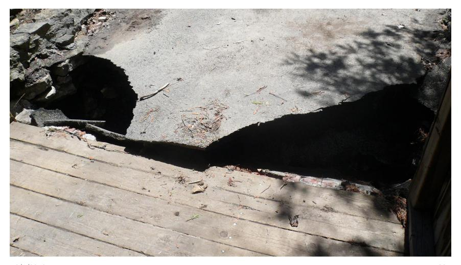
Picture 33 - Washed out concrete support slabs from the covered bridge - July 24/19
